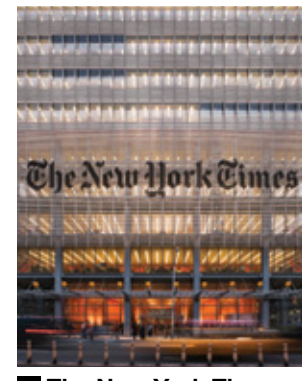
8 The New York Times Building Renzo Piano Building Workshop, in association with FXFWLE Architects 620 8th Avenue
