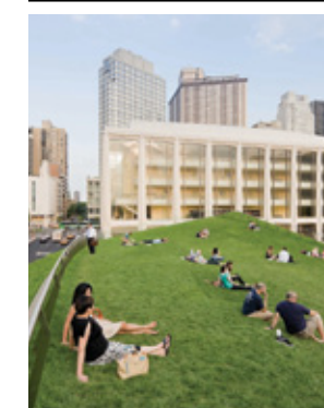
31 Hypar Pavilion Lawn and Lincoln Restaurant, Lincoln Center Diller Scofidio + Renfro in collaboration with FXFWLE Architects 142 West 65th Street
