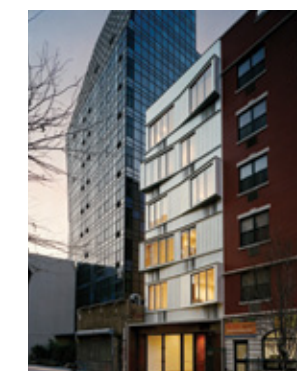
17 Switch Building nARCHITECTS 109 Norfolk Street
