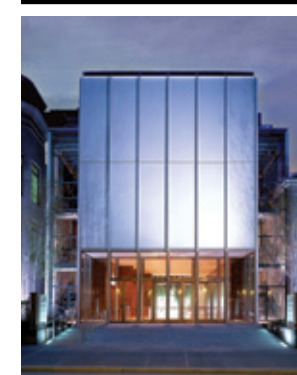
2 Morgan Library Renzo Piano Building Workshop/Beyer Blinder Belle Architects & Planners 225 Madison Avenue
